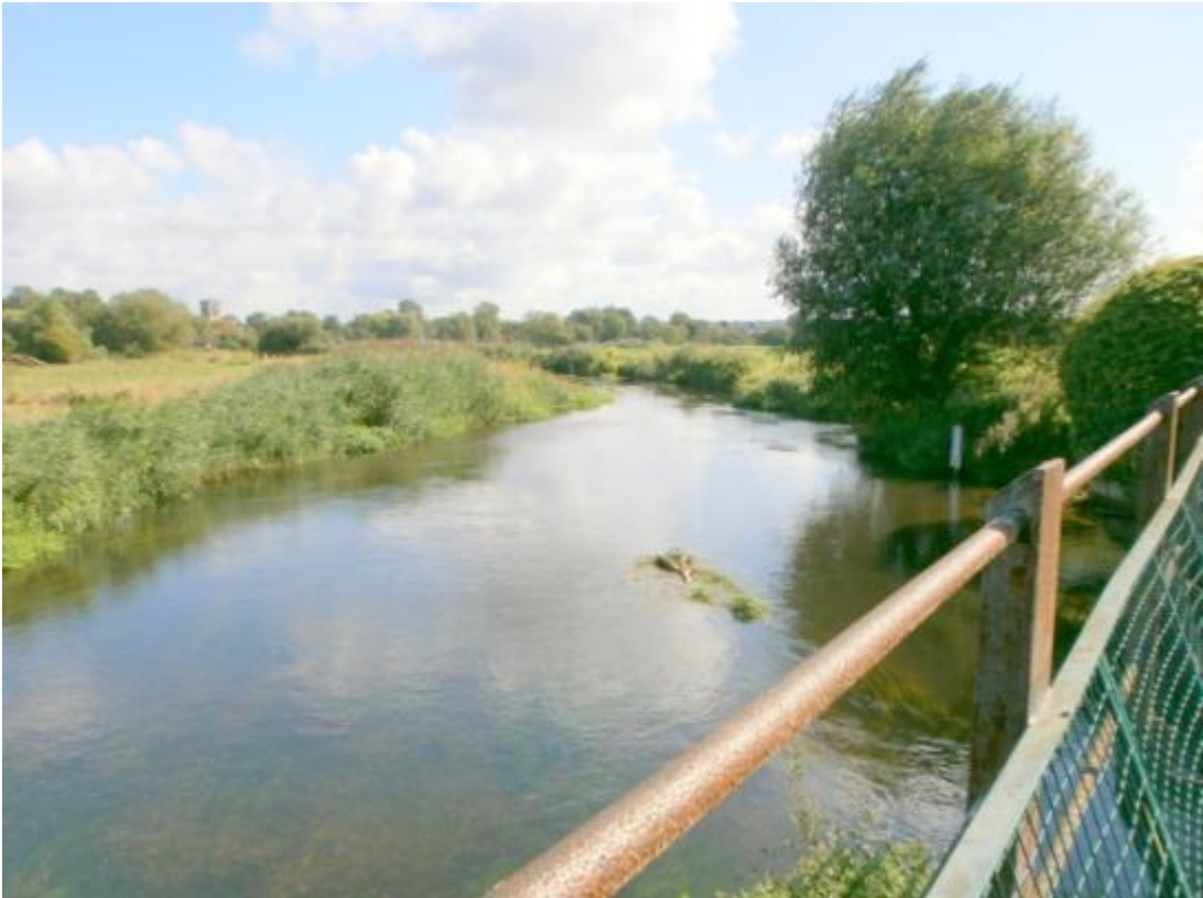
Figure 12. Looking upstream from Castlemain Tramway bridge
