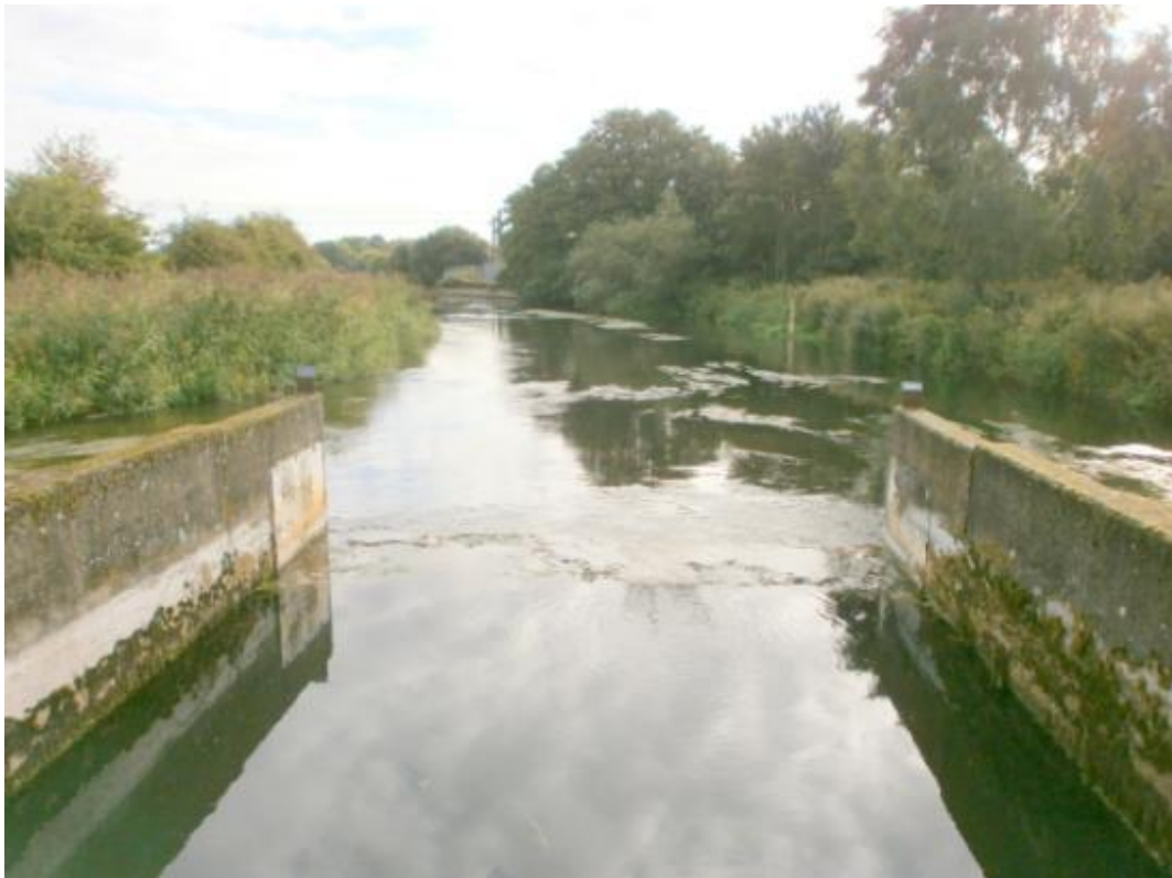
Figure 8. Upstream of Ringwood Weir.
